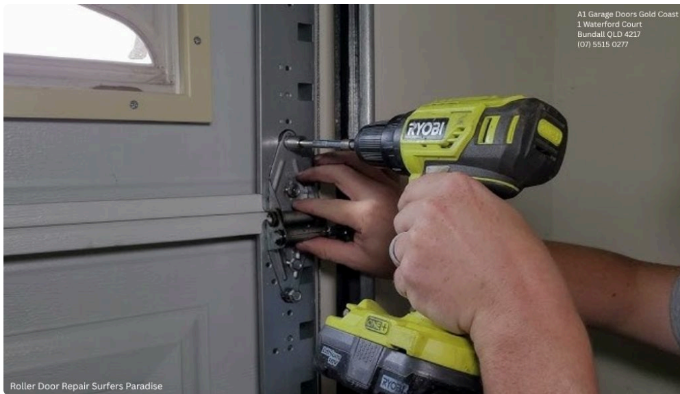
Roller Door Repair Surfers Paradise
